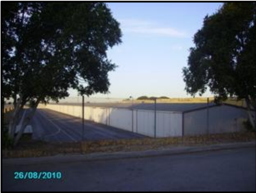
PHOTO 13: View of subject property from Alpine Way (looking south west)
