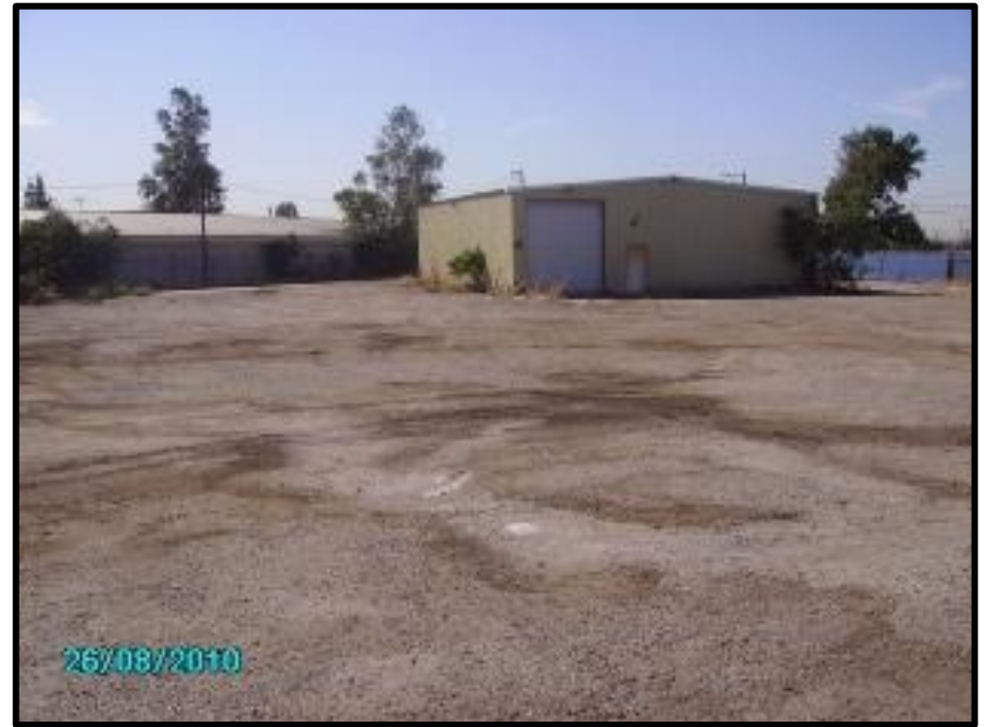
PHOTO 3.2: Construct second conventional hanger in helicopter area
