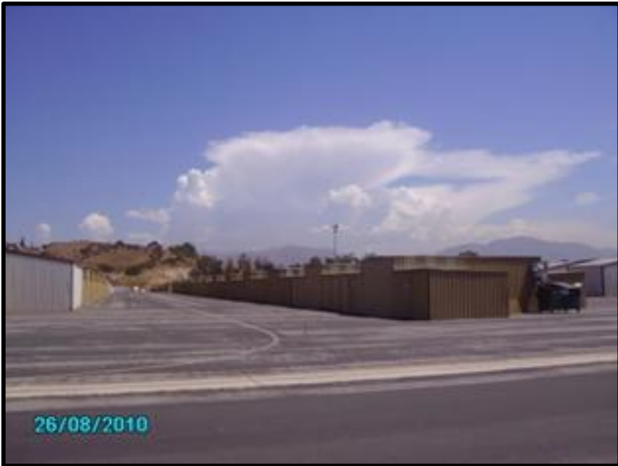
PHOTO 2.12a: Replace northeast county T-hangers
