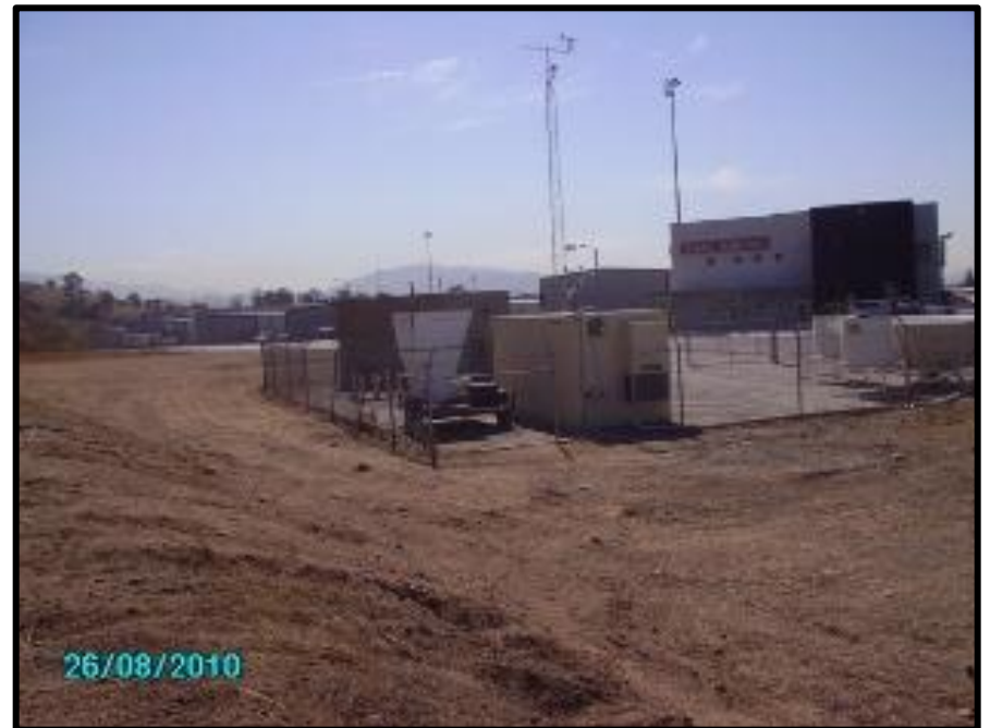
PHOTO 20: Poser and generator station on Airpark Way
