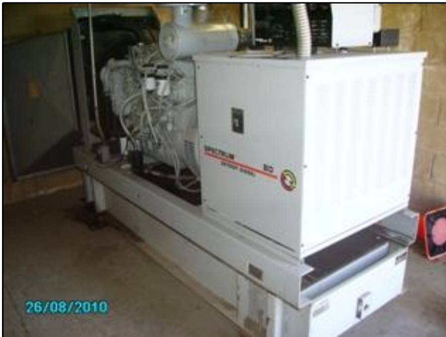
PHOTO 23: diesel generator in electric station
