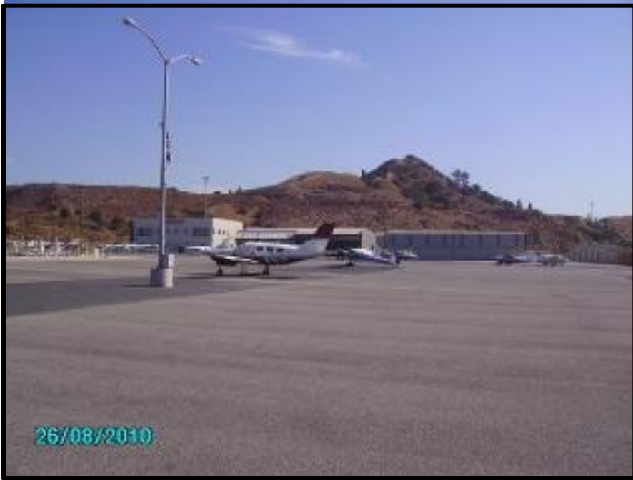
PHOTO 1.5: Construct Airport Apron
