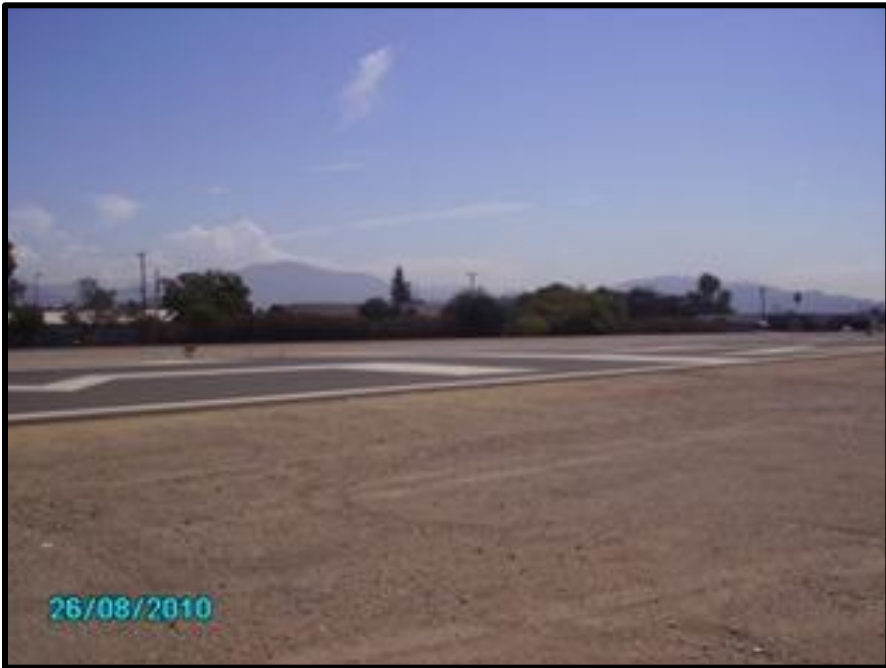
PHOTO 2.2: Relocate runway thresholds and painting non-precision markings
