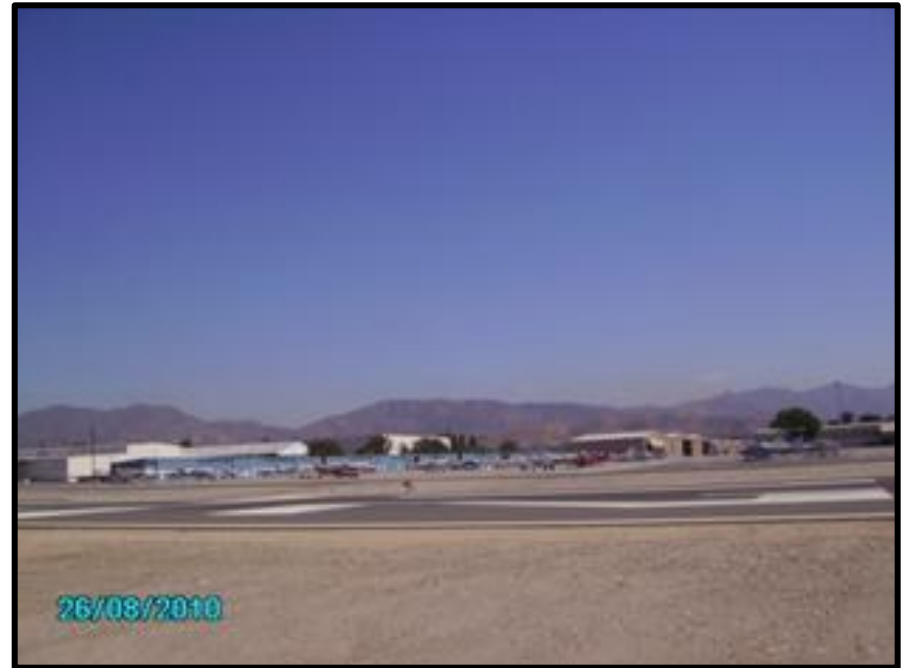
PHOTO 2.3: Construct runway 30 hold apron
