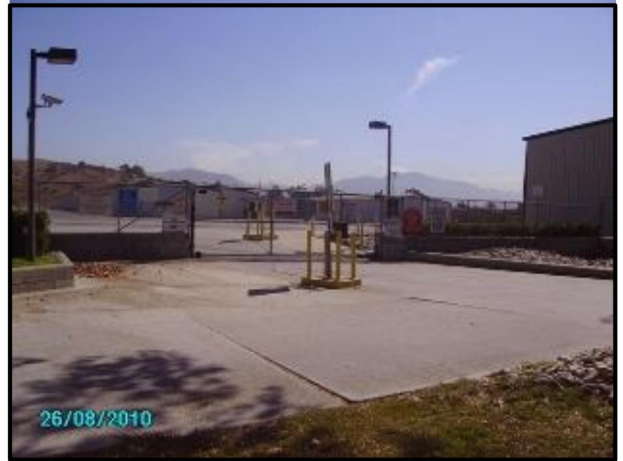
PHOTO 1.2: Perimeter fencing and "Penalty Box"
