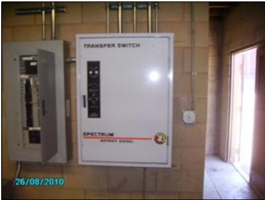
PHOTO 21: Switch gear in electric station
