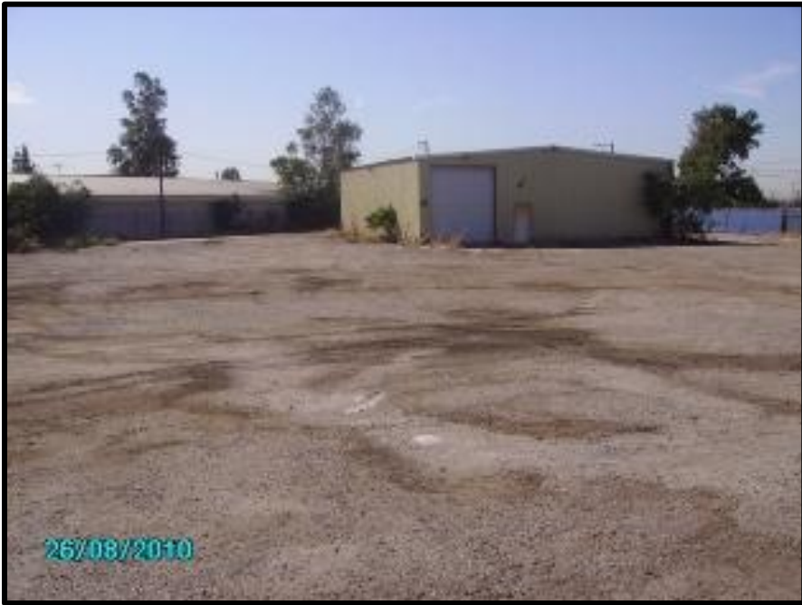
PHOTO 2.5: Construct new conventional hanger
