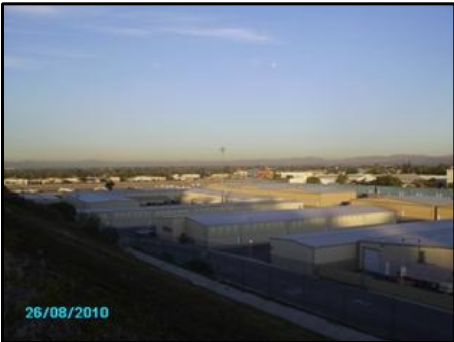
PHOTO 15: View of subject property from Alpine Way (looking northwest)
