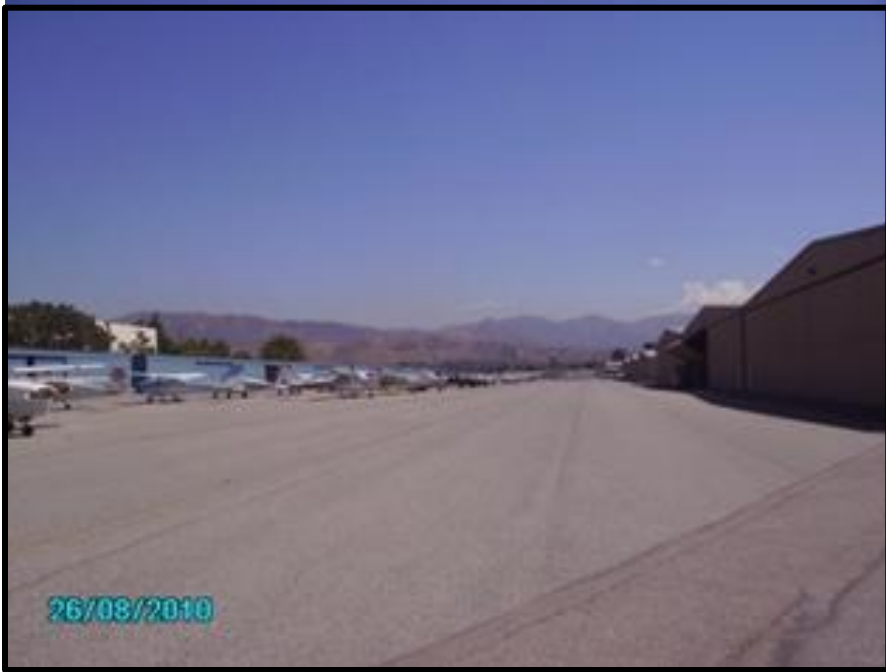
PHOTO 1.1: Repave and re-slurry aircraft parking
