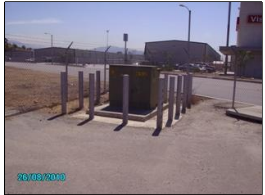
PHOTO 22: Power box n electric station
