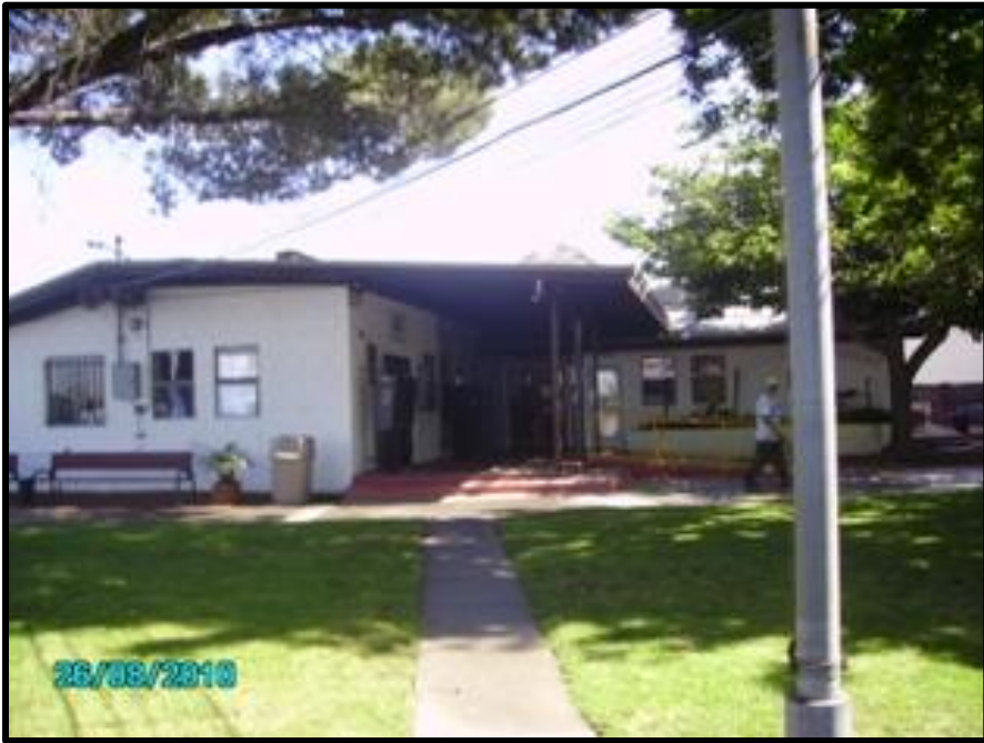
PHOTO 2.4a: Demolish existing terminal facility
