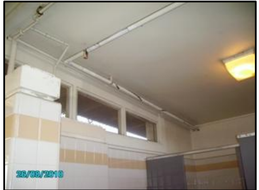
PHOTO 2.4d: asbestos covered pipes in restroom
