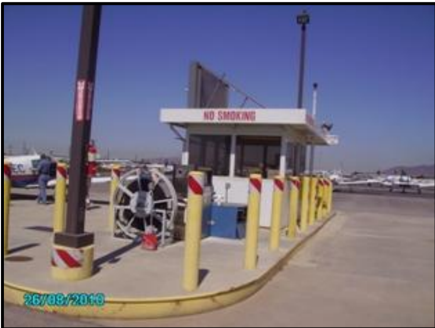
PHOTO 19: Dispenser island – no releases
